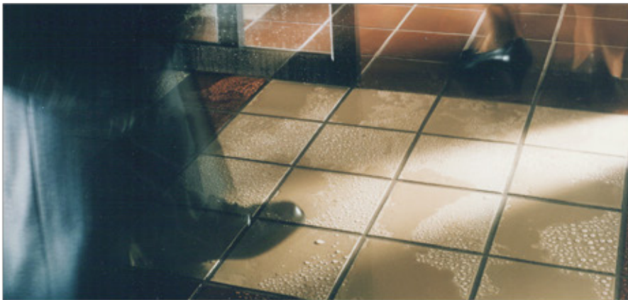
Photo above shows Metropolitan Ceramics Tile used in an entry platform. The image to the right shows a typical pass-through area.
